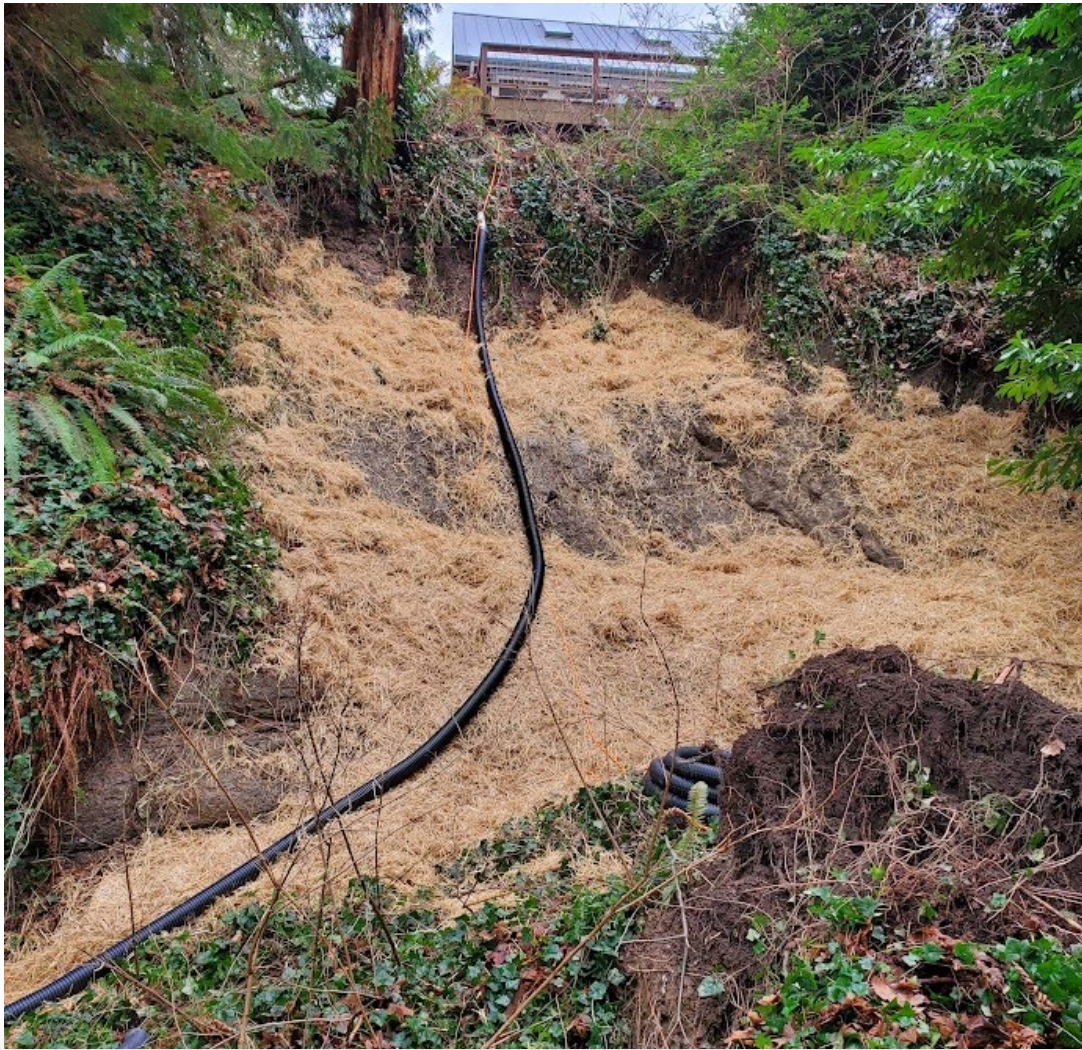
Landslide on Bainbridge Island – corrugated pipe duct tape to PVC outfall at crest
