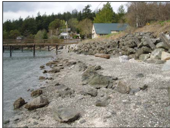
Figure 23. Toppling boulders over intertidal.
