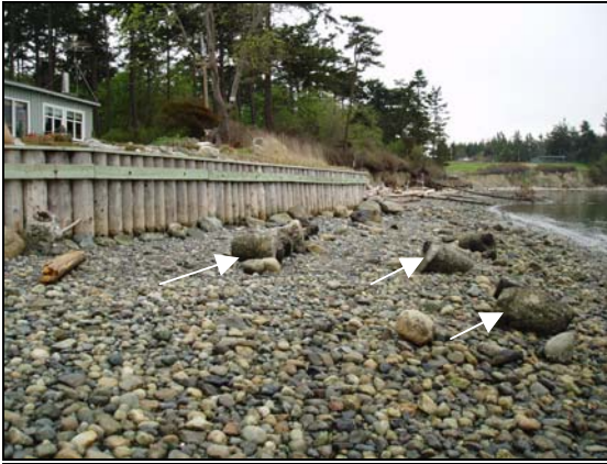
Figure 18. Aleck Bay soldier pile bulkhead.
