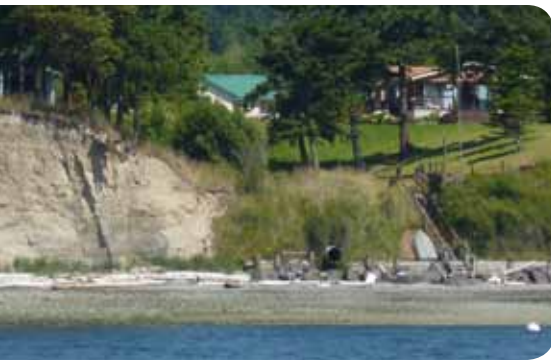
Stormwater infrastructure and runoff causes beach erosion and carries pollutants including sediments, toxins, and nutrients to the marine environment.
