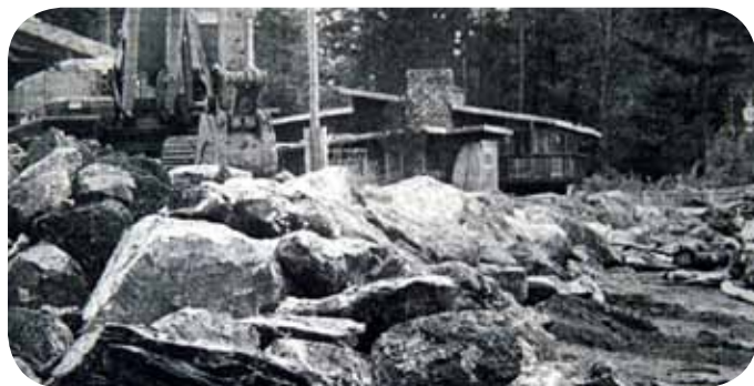
This example of soft shore restoration was completed in 1992 by Wolf Bauer. This beach located along North Beach, Orcas Island has a lot of exposure to high wind and wave energy. The restoration project made the shoreline healthier for fish, wildlife and people while also protecting the homes from erosion. Before photo courtesy of Wolf Bauer. After photo, taken 12 years later, by Jim Johannessen, Coastal Geologic Services.
