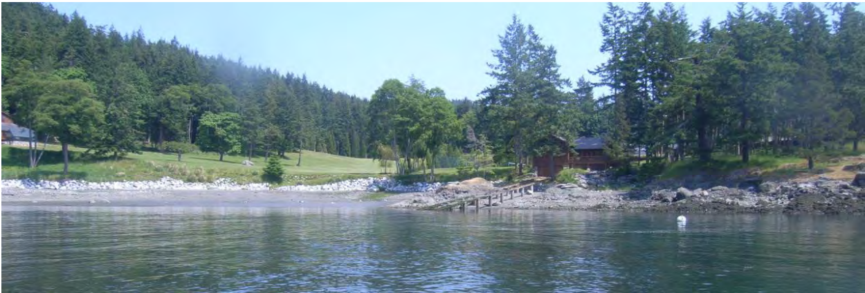
SE Blakely Island. Highest fish use region and shoreform. Pocket beach, relatively long structure. Note: unpermitted structure and additional, newer unpermitted armor to the south (left in photo). Active land use case with San Juan County.
