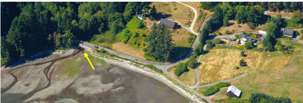
Tier 1. Olga road, Buck Bay Orcas High fish use region and shoreform and top priority stream. County road/bridge. Note: bridge installed recently to replace armor/fill/perched culverts and improve tidal hydrology.
