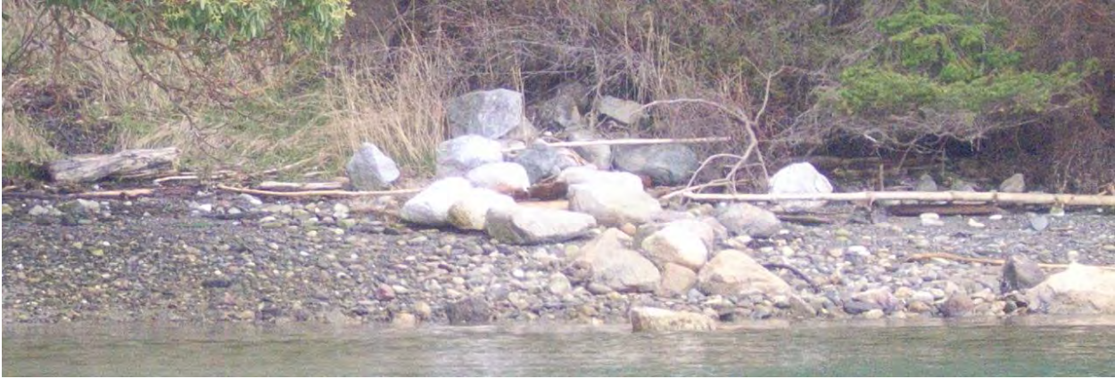
Tier 1 Groin Removal, Turn Point, San Juan High fish use region and shoreform.
