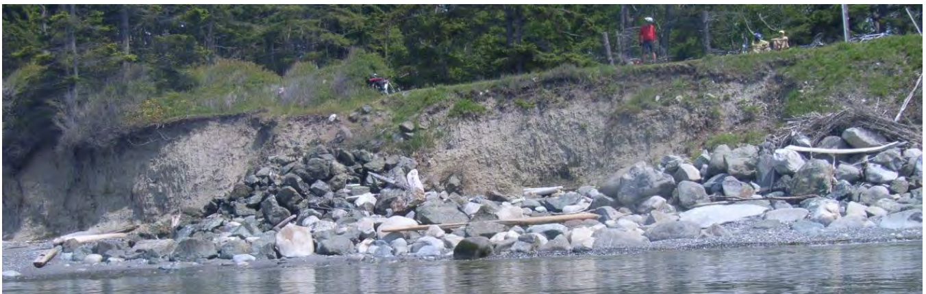
MackKaye Harbor Rd., S. Lopez County road. Highest priority fish use region and shoreform. Documented forage fish spawning beach downdrift of bluff. Extensive length. S. of County Park.
