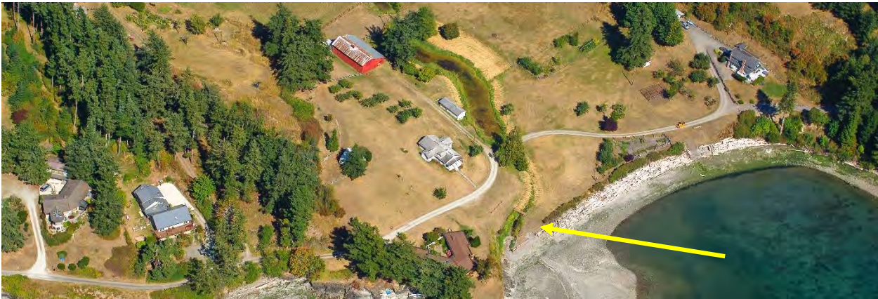
Tier 2. SE Eastsound, Orcas. High priority fish use region and fish bearing stream.
