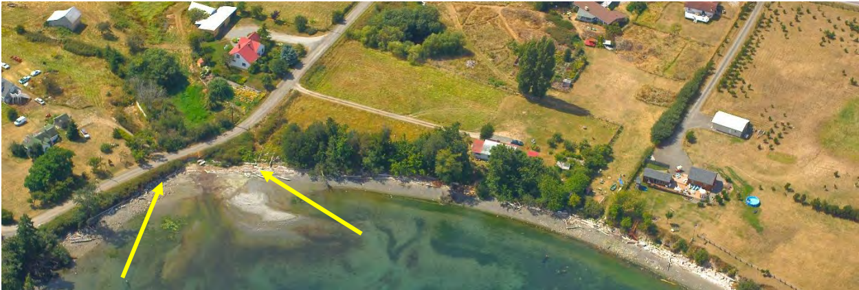
Tier 2. Mill Creek Road, Griffin Bay, San Juan Island High fish use region and fish bearing stream. Culverts associated with a county road.
