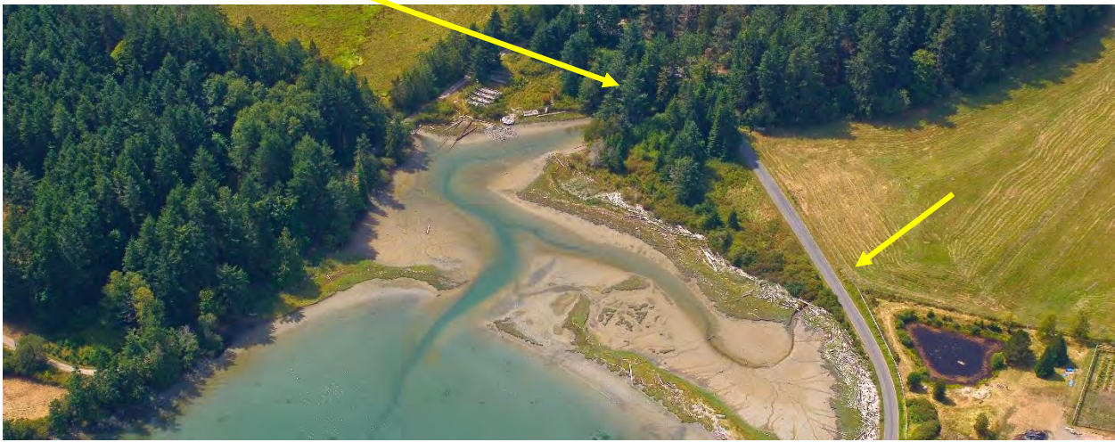
Squaw Bay Road, Squaw Bay, Shaw. Fish bearing stream. Culverts associated with a county road.
