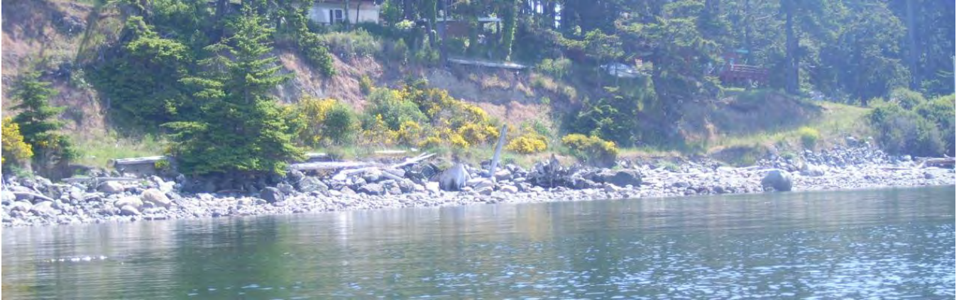
Islandale, MacKaye Harbor, Lopez. San Juan County Public Works and private ownership. Dock, boat ramp, a shoreline road and multiple groins as well as armor. Highest priority fish use region and high fish use shoreform.
