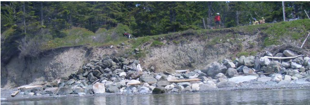
MackKaye Harbor Road, Agate Beach, Lopez. Highest fish use region and shoreform. Pocket beach/bluff. Forage fish spawning down drift. County road and private shoreline ownership.
