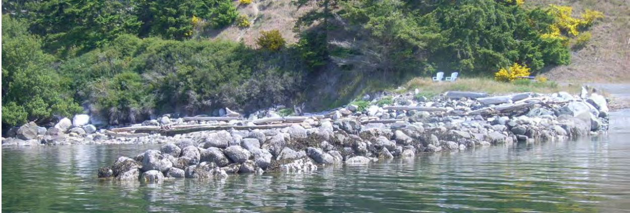
Tier 1. Groin Removal Islandale, MacKaye Harbor, Lopez. San Juan County Public Works shoreline parcel (includes shoreline road, armor, dock, ramp, multiple groins). Highest priority fish use region and high priority fish use shoreform.
