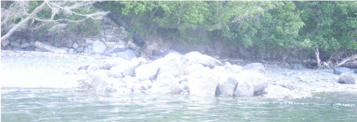
Tier 1. Groin removal Mud Bay Lopez High fish use region and shoreform. Documented forage fish spawning site. Priority bluff.
