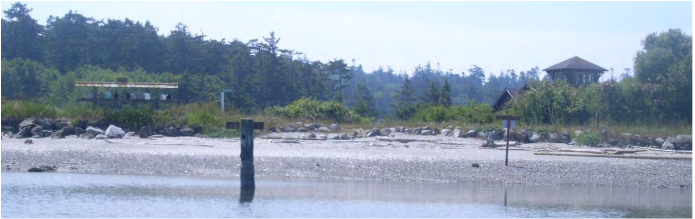
MacKaye Harbor Rd. Barlow Bay, Lopez County road, private shoreline ownership. Documented forage fish spawning site. Extensive length. Also a tidal barrier in multiple locations.
