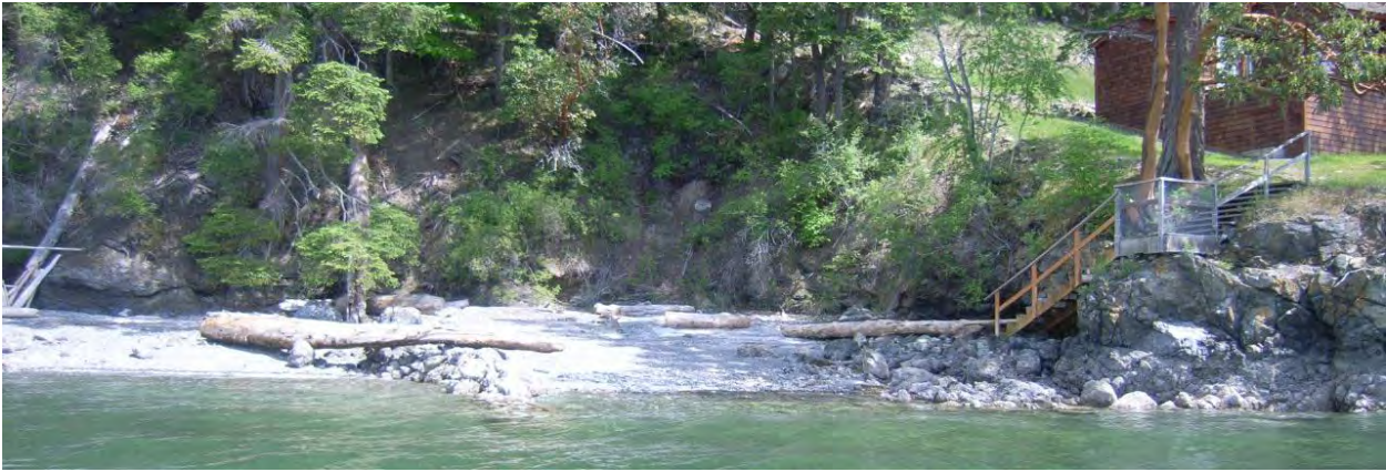
Tier 1 Groin Removal, Eastsound, Orcas. High priority fish use region and shoreform.
