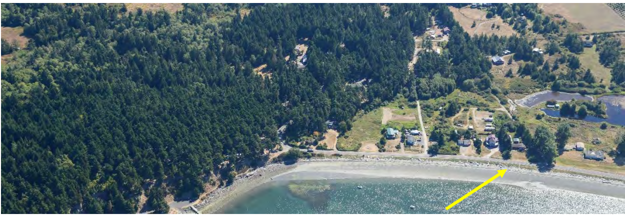
Tier 1. MacKaye Harbor Road, MacKaye Harbor Lopez. Highest priority fish use region and shoreform. Culvert(s?) associated with county road.
