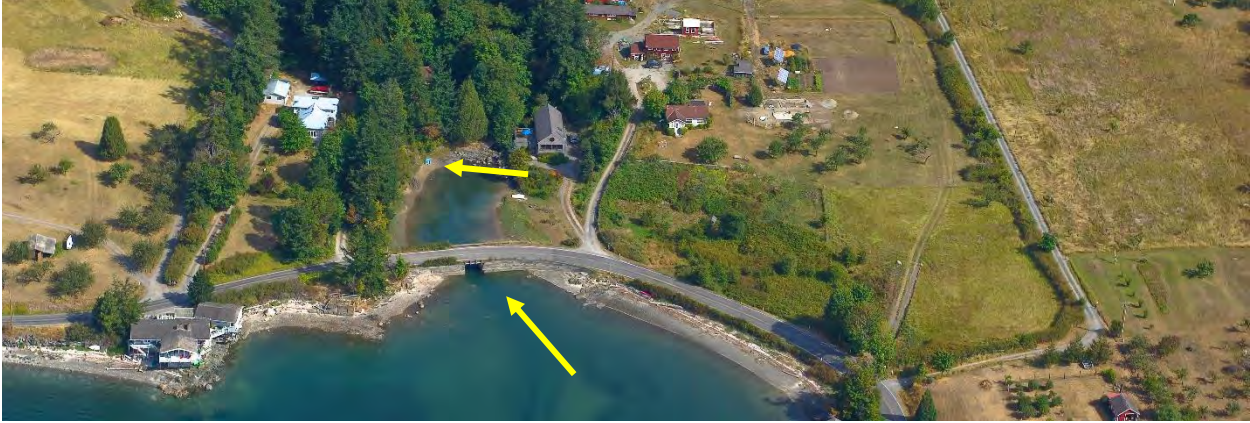
Tier 1. Deer Harbor Road, West Sound Orcas. High priority fish use region and fish bearing stream. County road/bridge, plus private barrier upland.
