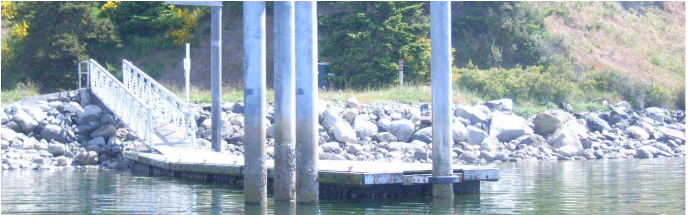
Islandale, MacKaye Harbor, Lopez. San Juan County Public Works Ownership. Dock, boat ramp, a shoreline road and multiple groins as well as armoring. Highest priority fish use region and high fish use shoreform.
