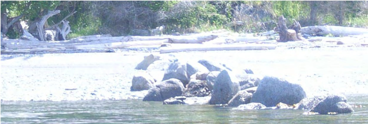
Groin removal, SW Lopez. High fish use region.
