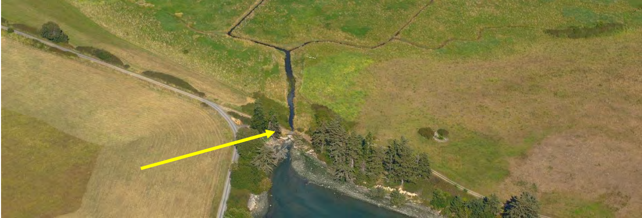
Tier 2. Davis Bay, Lopez Island. Highest priority fish use region and large area. Tide gate associated with a private road. Note: additional barrier from a county road at upper edge of wetland complex. SJC Land Bank and Preservation Trust easements in area.
