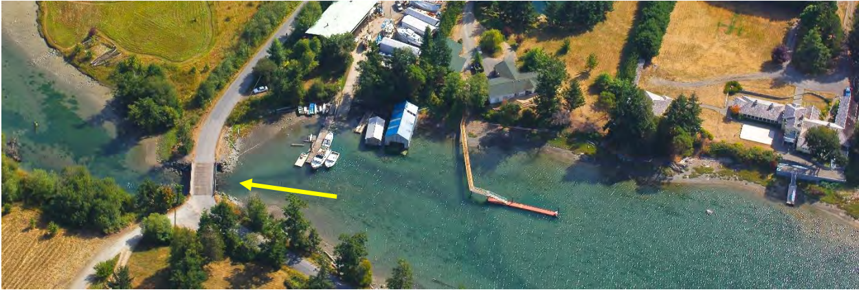
Tier 1. Channel Road, Deer Harbor, Orcas High priority fish use region and priority region. County road/bridge. Note: larger span bridge installed in 2016 that improved tidal hydrology.
