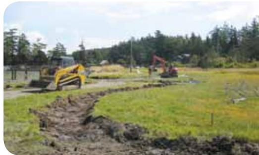
*During: New channels were created to open the salt marsh to marine waters.*
